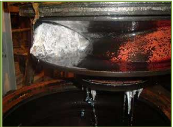
Figures 4.1.1.a & 4.1.1.b – Details the typical extent of a blockage in pump impellers prior to implementing new intelligent control regime.
