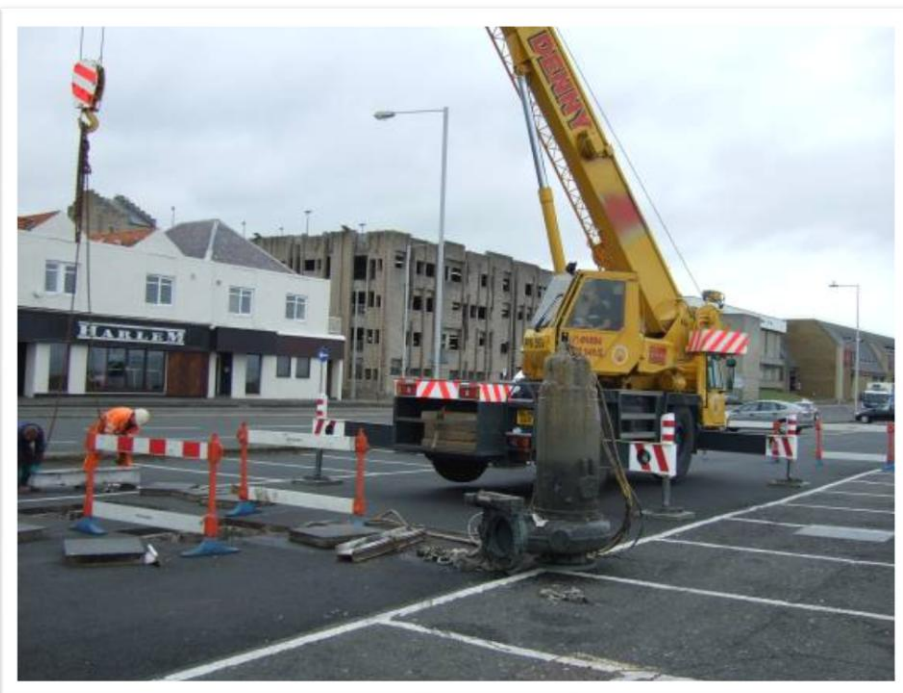
Pump lift and clean
